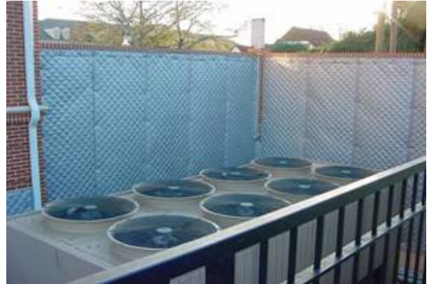
Brick wall attachment of HUSH FLEX™ panels.
