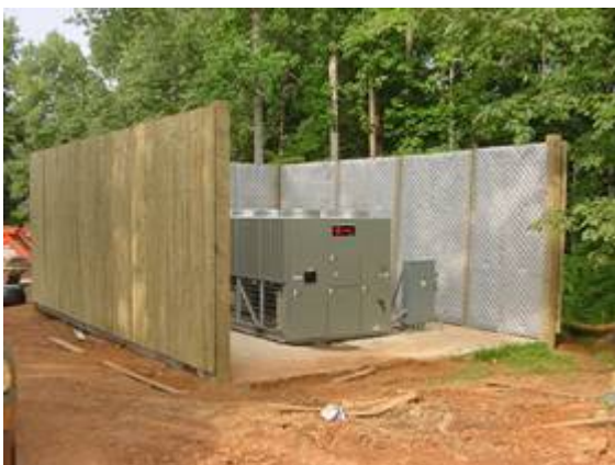
HUSH FLEX™ panels attached to wood planking fence.
