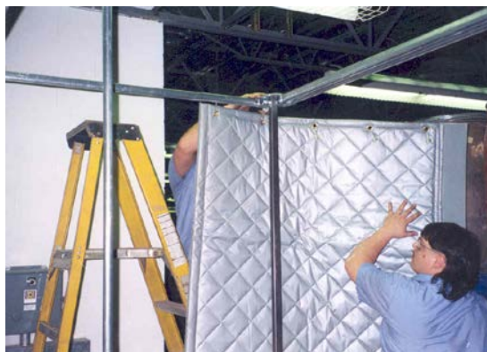
ABAC-111N panel with 4" corner strip hung on roller trolley and track system.
