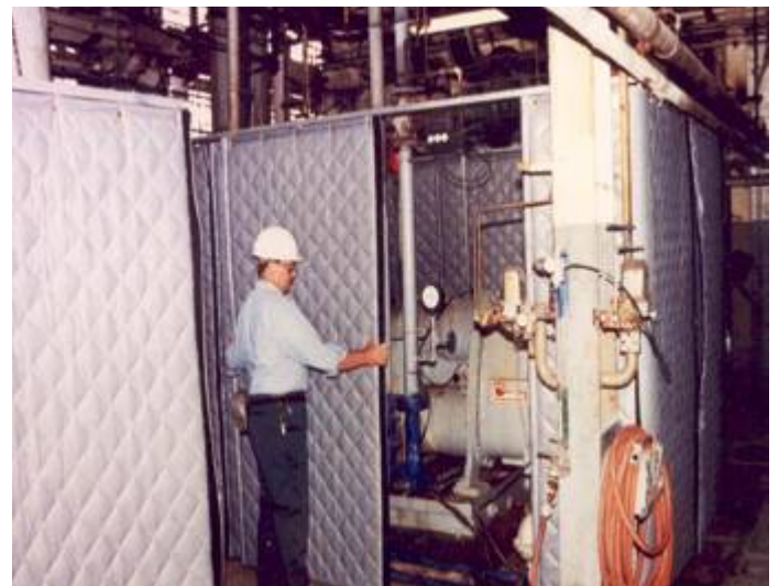
Typical double track design sliding panel access for compressor enclosure.
