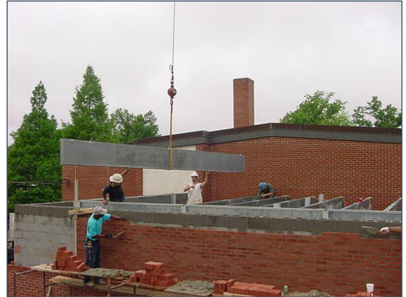
Installation of HUSH GUARD™ Roof Baffle Splitters
