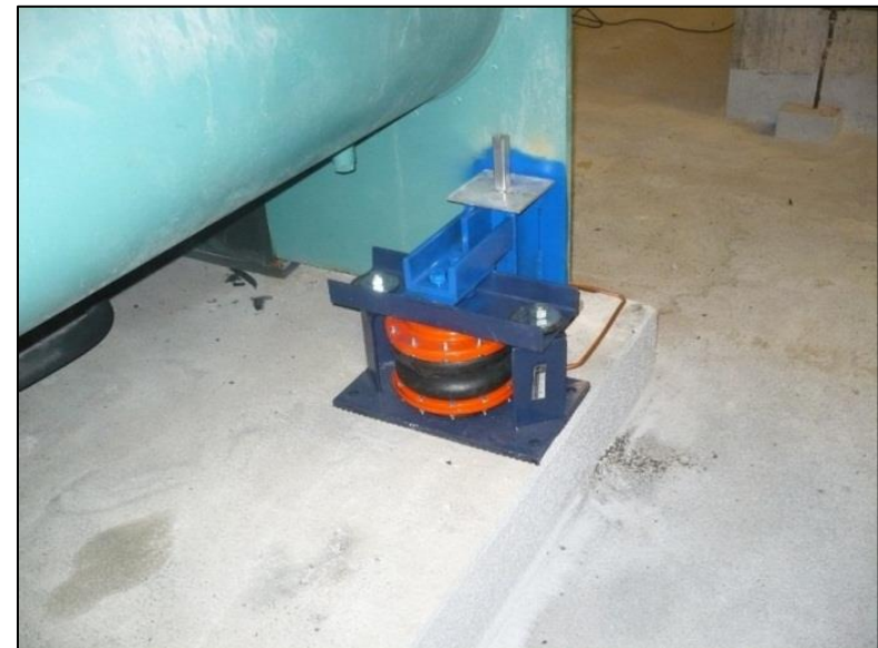
HUSH MOUNT™ Pneumatic Isolation System
