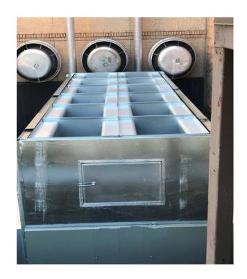
Hush Duct<sup>™</sup> To achieve the attenuation needed to adequately satisfy the neighbor complaints, a Summit System<sup>™</sup> chiller enclosure was created using Hush Duct<sup>™</sup> intake and discharge silencers and Hush Guard<sup>™</sup> panels.
