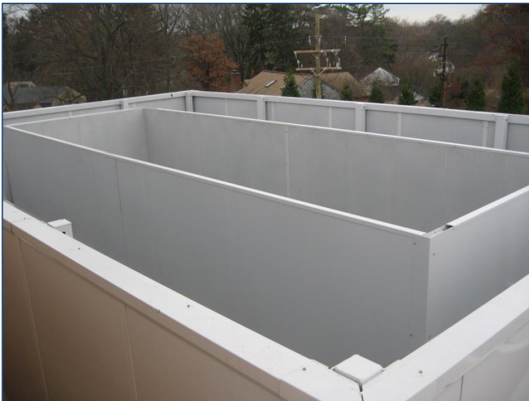
Integrated Condenser Fan Discharge Plenum
