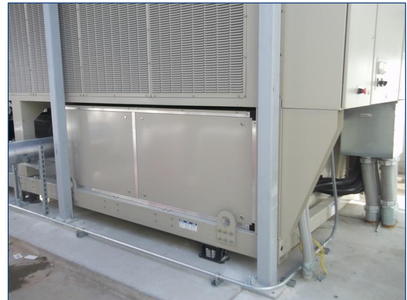
Independently Supported Steel Framing for Discharge Stacks
