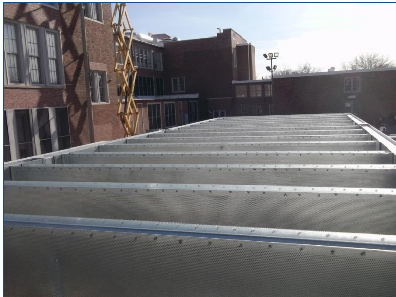
Baffle Close-Up Showing School Building Classrooms in Background
