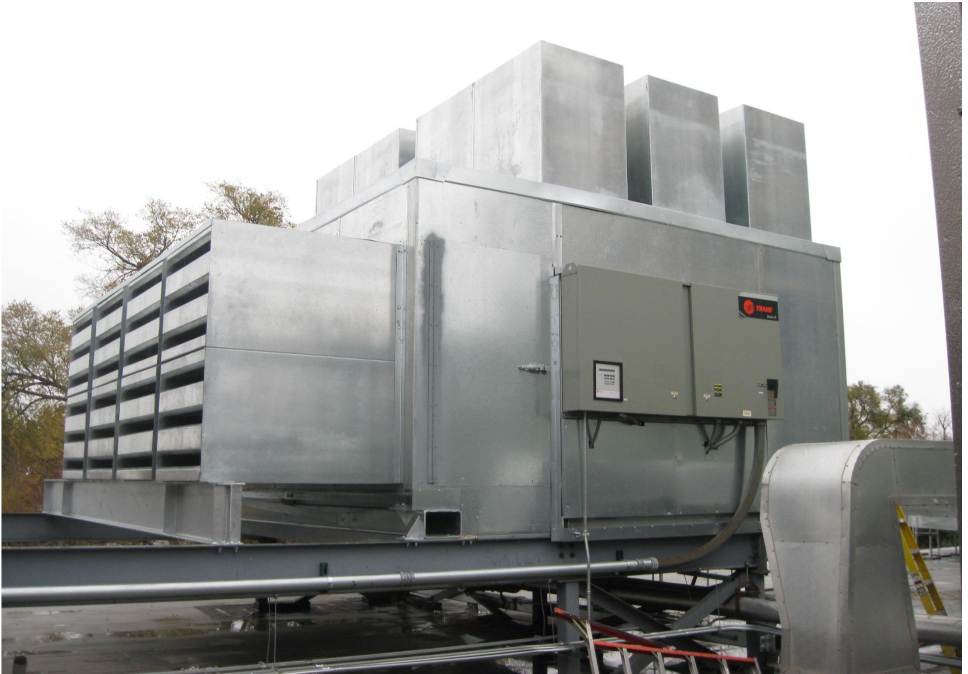
Finished Ultimate™ System with 7' Long HUSH DUCT™ Intake and Discharge Silencer Banks
