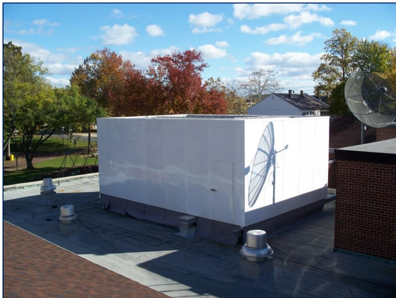
Finished Supreme™ System Rooftop Chiller Enclosure
