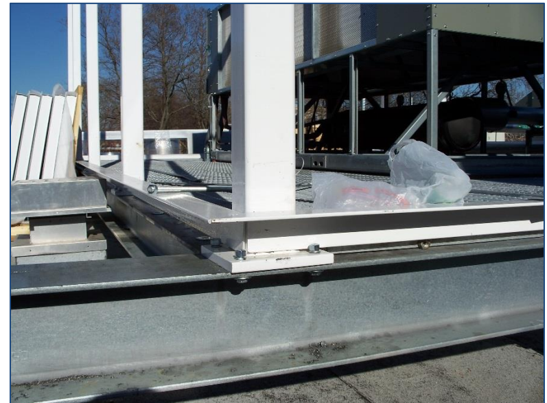
Column Tie In At Dunnage Steel Support
