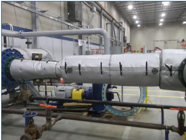
Finished HUSH COVER™ Removable Blanket Installation
