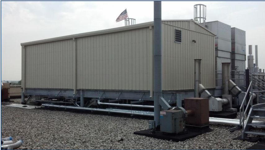
Penthouse Acoustical/Weather Enclosure
