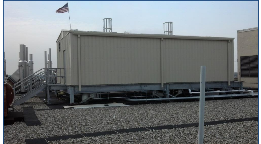
Dunnage Supported Finished Ultimate™ System Enclosure
