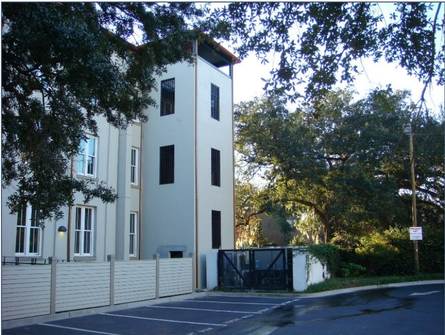
Untreated Chiller Next to Condominium Building
