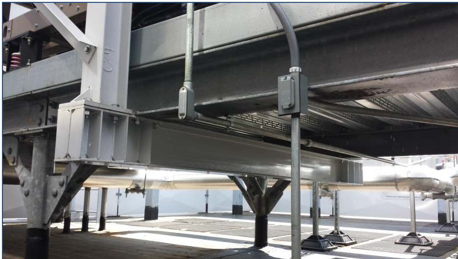
Independent Underbeam Mounting of Chiller Discharge Acoustical Stacks
