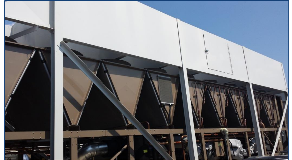
Condenser Fan UnitaryPlus™ Discharge Stacks
