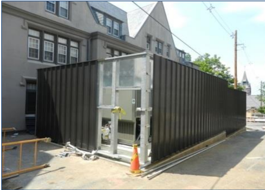
Partially Erected Perimeter Screen™ System Chiller Enclosure
