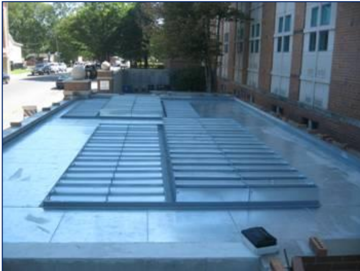
Chiller Enclosure HUSH GUARD™ Roof with HUSH DUCT™ Banks for Airflow
