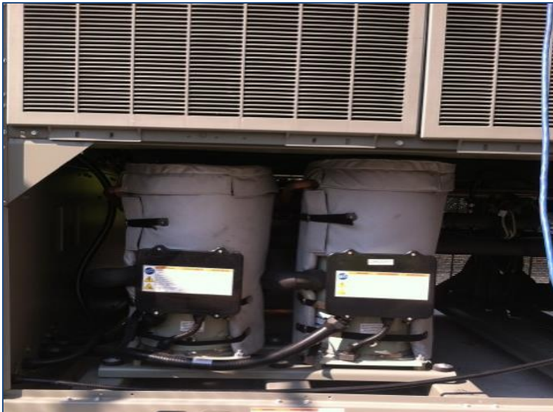
Standard™ “SL” System HUSH COVERS™ for Scroll Compressors
