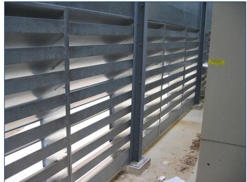
Inside View of HUSH DUCT™ Integrated HDAL Acoustical Intake Louvers
