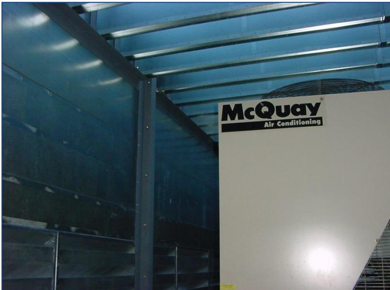
Inside View of Ultimate™ System Discharge Roof Baffles
