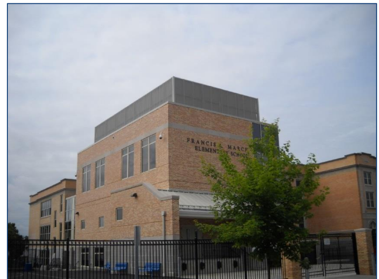
Outside View of Finished Premium™ “OF” System Chiller Enclosure
