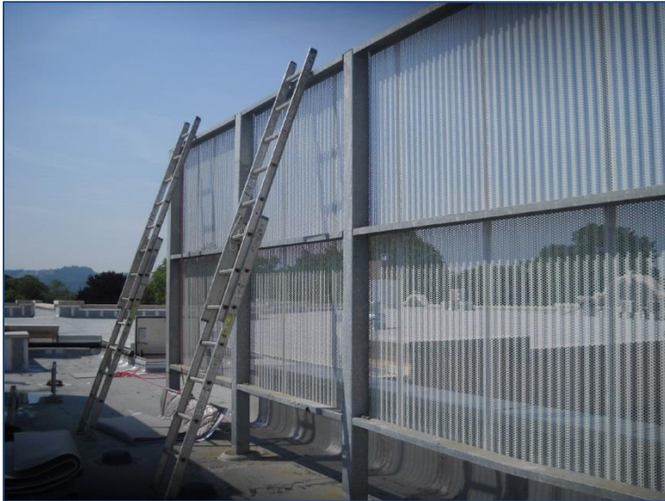
Untreated Chiller Visual Screen
