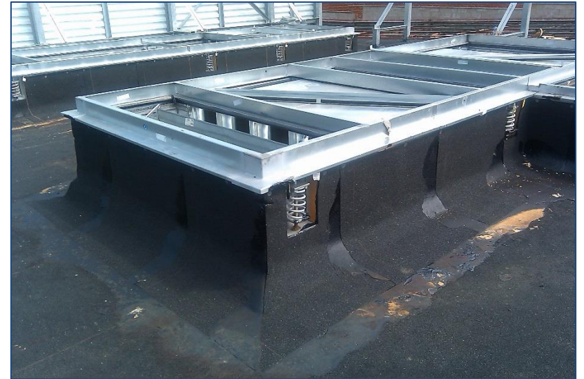
Acoustical Curb Waiting for RTU Pick
