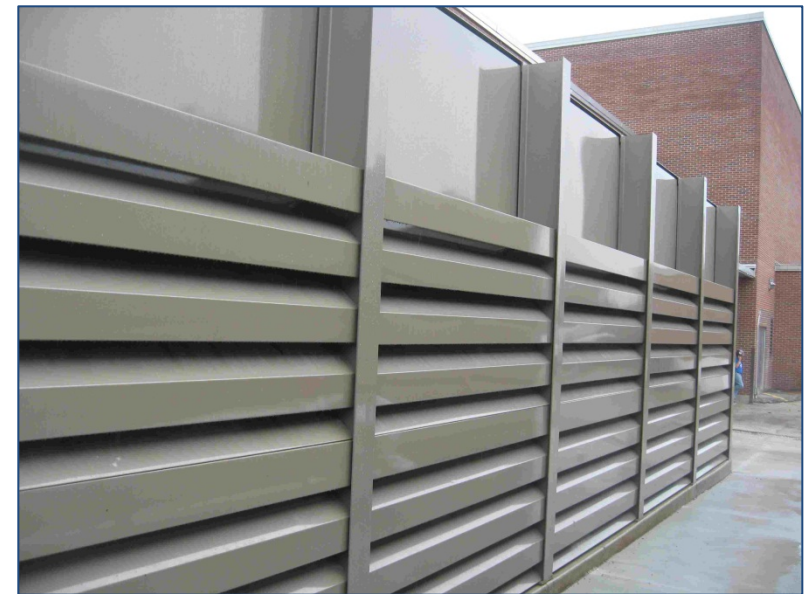
Close-Up of HUSH DUCT™ Acoustical Louver HDAL Intakes
