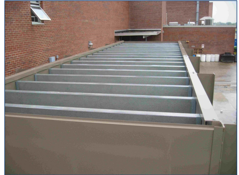
Top View of UnitaryPlus™ Condenser Fan Discharge Stack
