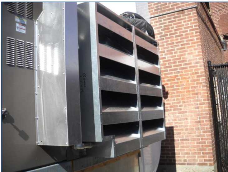
HUSHCORE™ UnitaryPlus™ Splitter Baffles
