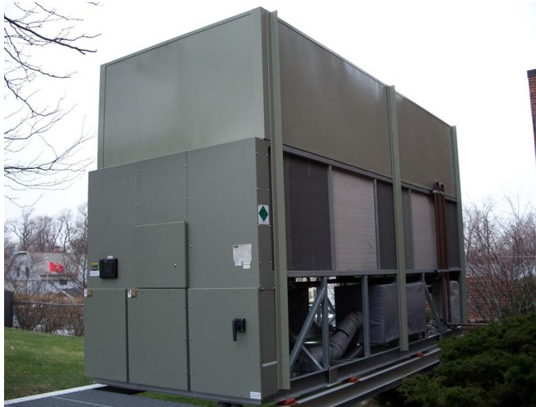
1. Locate chiller unit framing to which the 3"x3" angle irons (supplied with HUSHCORE™ *Unitary*™ System) may be mounted. Half of the lengths of supplied angle iron should be installed and evenly distributed on one side of the chiller unit and the other half on the other side. None are required on the ends of the chiller.
