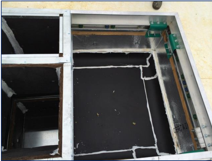
HIC-DS-41 PLUS™ System with HIC-2 Isolation Curb & DS-41 in-curb treatment
