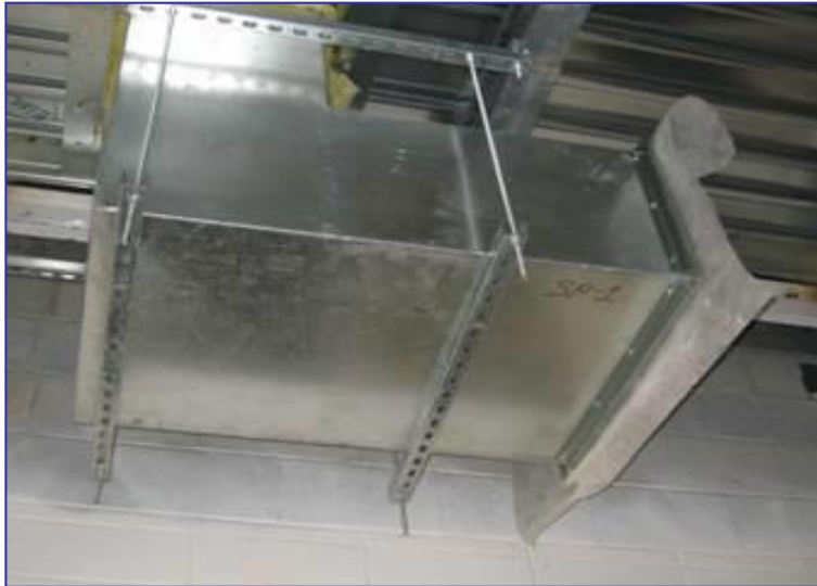
HUSH DUCT™ silencer mounted directly below roof deck opening to minimize in-duct noise
