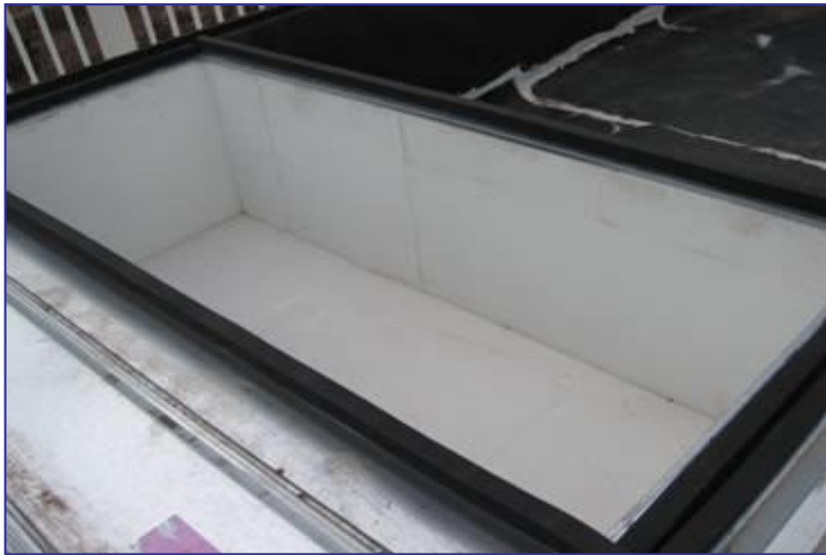
Model HUSH LINER™ HLM-100-H Fiber-Free, Non-Fiberglass Duct Liner
