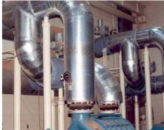
HUSH WRAP™ built-up component system on blower piping in a wastewater treatment plant.
