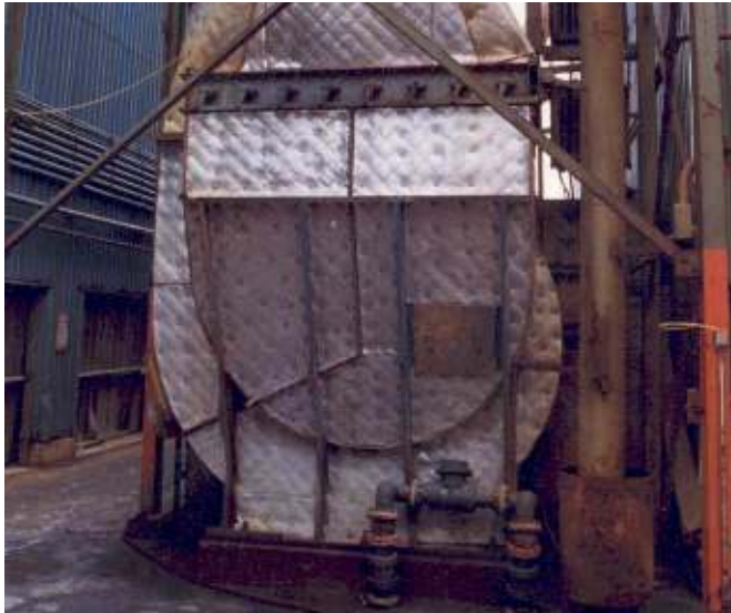
HUSH WRAP™ composite material type LVQ-210-LAG installed using stick pin fasteners on outdoor fan installation.
