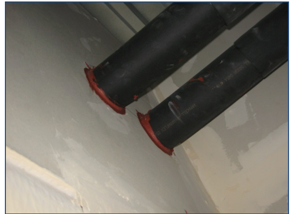
Fire-rated wall pipe penetration using HUSH SEALANT™ HSAC-FS-100
