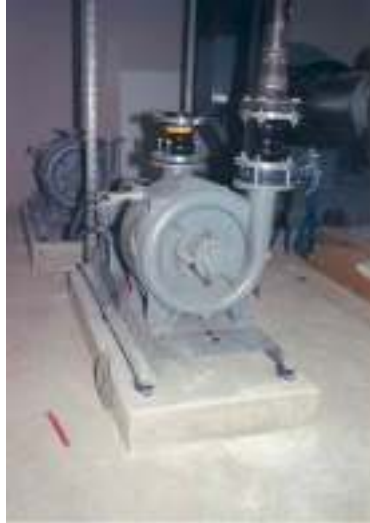
Style HJ-TS twin sphere flex connector for centrifugal pump installation.
