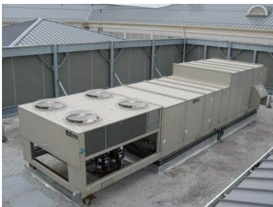
Rooftop sound barrier wall for HVAC unit
