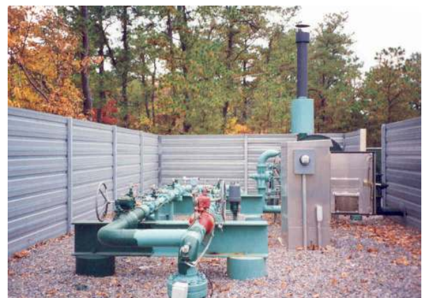
Metering station sound barrier wall
