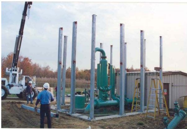
Structural steel columns are erected.
