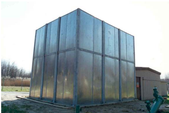
Type HG-400 acoustical panels erected in the structural framework.
