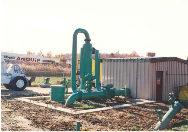
Foundation with anchor bolts for columns.
