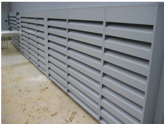
Close-up view of HUSH DUCT™ HDAL-1206 banked modules.
