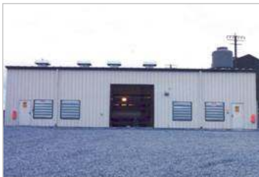
Blower building air intakes with HDAL-1209 Acoustical Louvers
