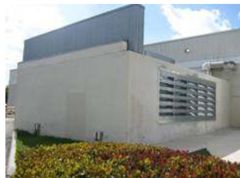
Dade County Compliant Hurricane Grade HUSH DUCT™ HDAL Louvers
