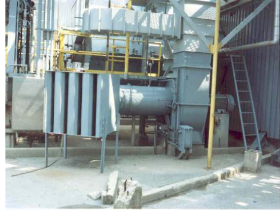
Industrial forced draft fan with model 3RL rectangular inlet silencer, support legs and transition.
