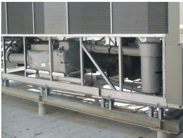
HUSH COVER™ on air cooled screw chiller suction lines, compressor, discharge line and oil separator.
