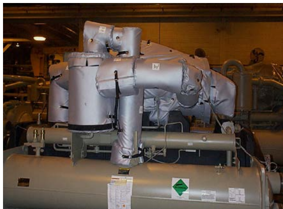
Liquid cooled screw chiller noise is tamed using HUSH COVER™ model HC-500S-1"
