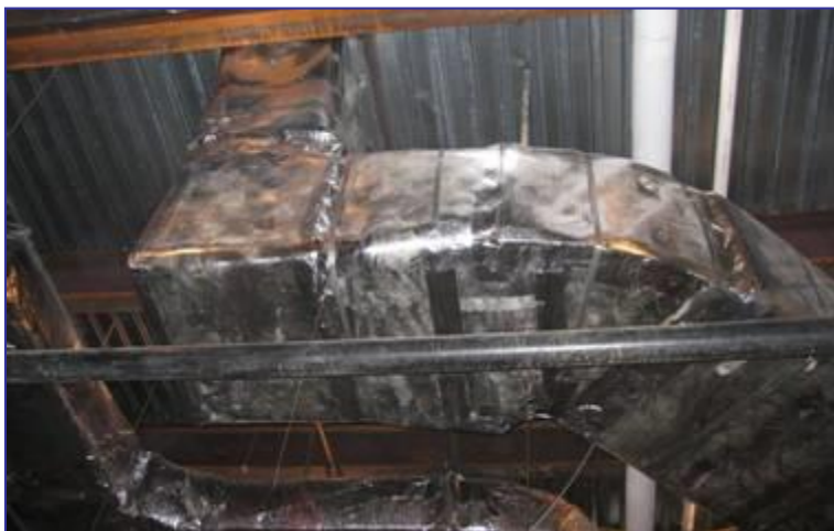
Supply drop with BARRICADE™ System external acoustic lagging
