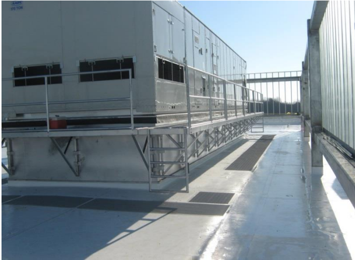
WHISPER™ Type “P” solid bottom plenum curb with segregated SA & RA divider
